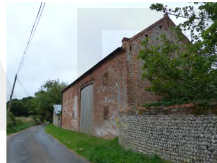
Converted threshing barn near Edgefield Old Rectory
