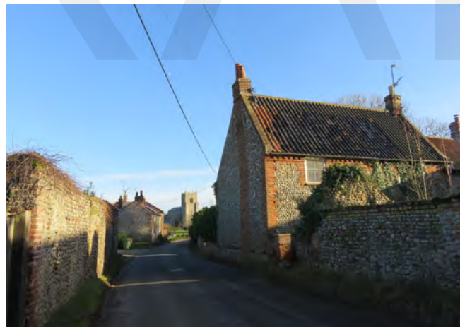
Typical vernacular dwellings along Blakeney Road flanking a view of the church
