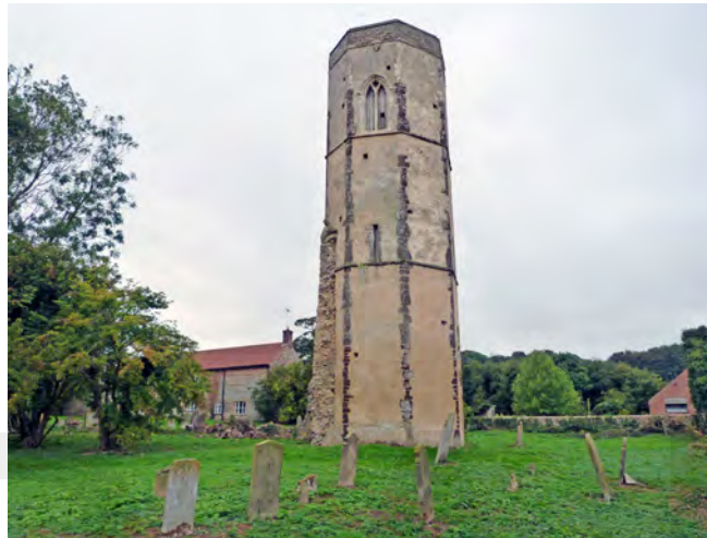
Stone used at the former Edgefield Church
