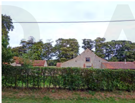
Converted farm buildings at Swan Lodge
