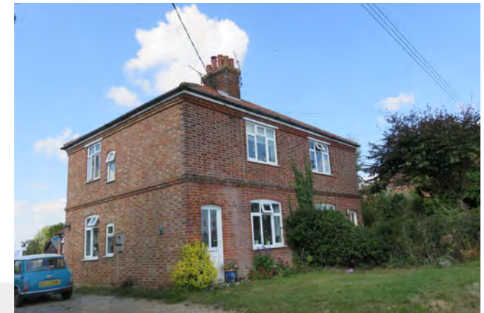
One of the pairs of semi-detached houses in Edgefield that is a rare example of pre-war parish council housing
