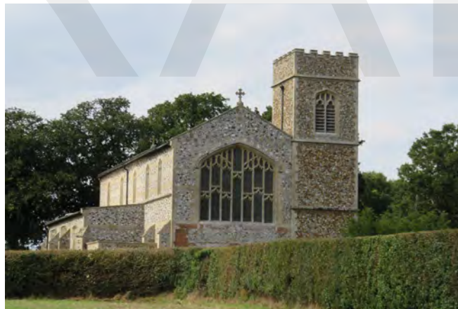
The rebuilt church at Edgefield
