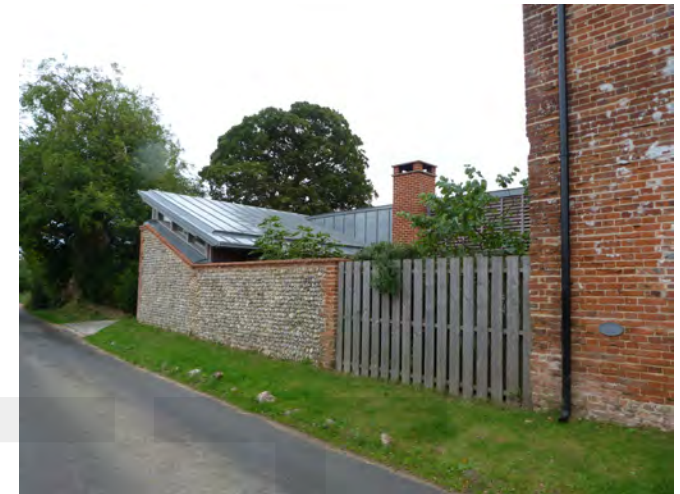
Zinc roof together with more traditional brick and flint to an extension to a barn
